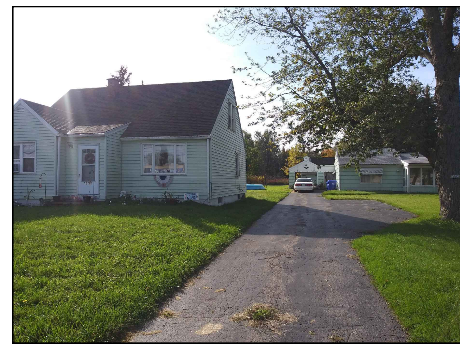
FROM NORTHWEST CORNER OF PROPERTY
