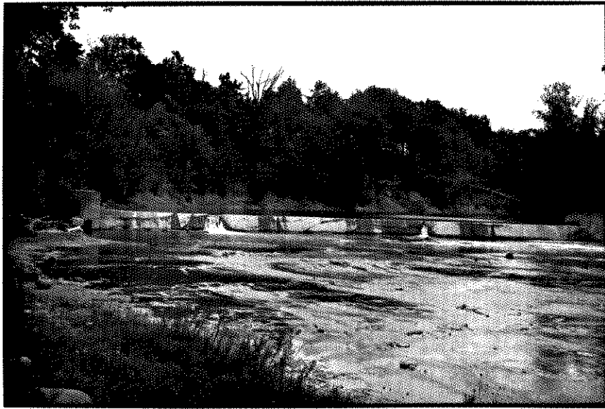
Photo No. 23. Elma Dam upstream of Bowen Road near mile 10.2. Note shale on right bank upstream of the dam.
