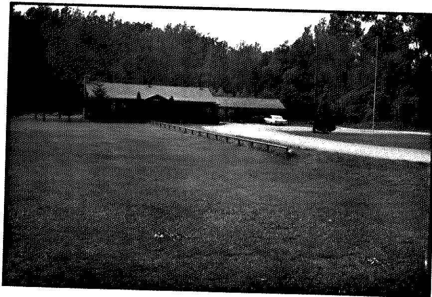
Photo No. 34. Elma Conservation Club near mile 14.8. Although the club house is high, the property near the creek is subject to flooding.
