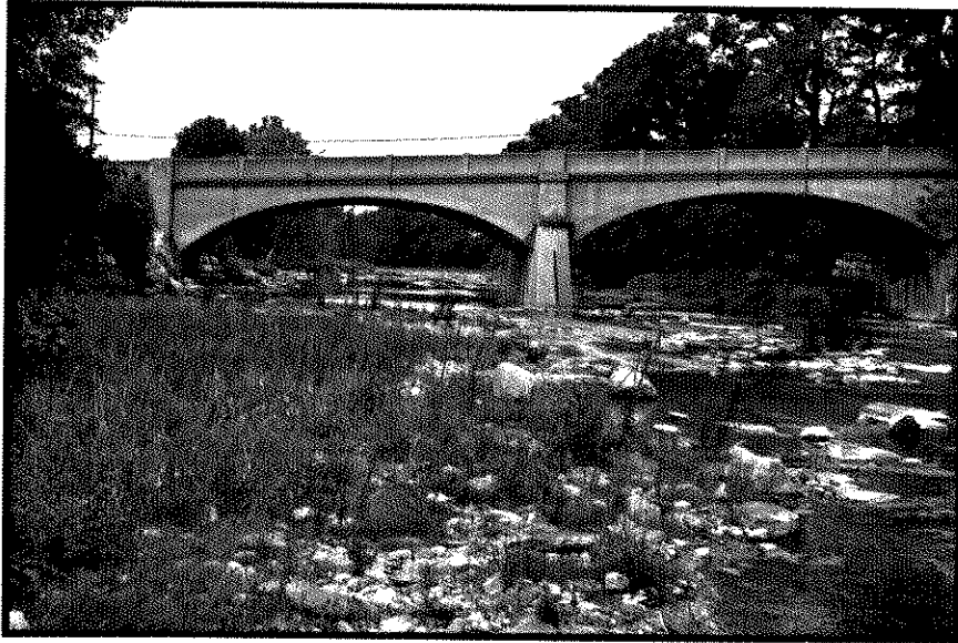
Photo No. 19. Looking downstream at Borden Road bridge showing rock channel bottom and shoals.
