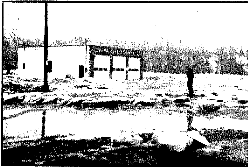
Photo No. 12. The new Elma Fire Hall during the March 1962 flood. The floor was covered by 8 inches of water.
