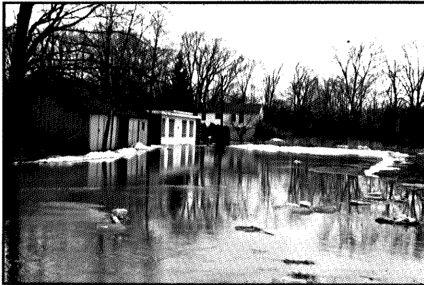
Photo No. 14. Rear of Sunday School addition during the March 1962 flood. Addition now being used for regular school classes. The addition had 4 inches of water on the first floor.
