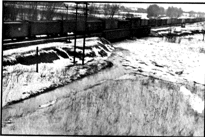
Photo No. 8. Looking at upstream side of the N.Y.C. R.R. bridge from Indian Church Road. This flood took place during the 1950's.
