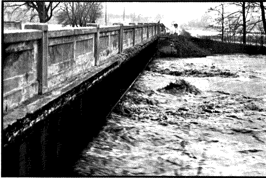
Photo No. 7. Looking south from the north abutment at the downstream side of the Transit Road bridge during the March 1955 flood.
