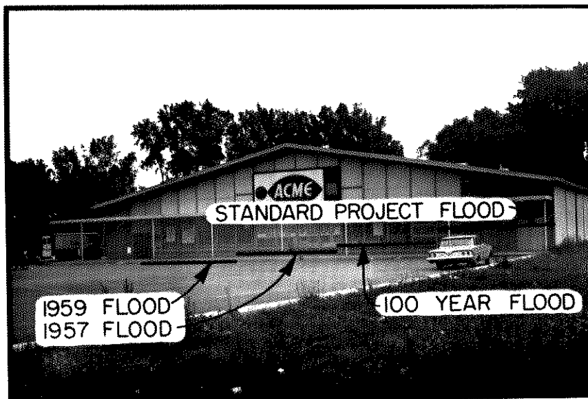
Photo No. 28. Supermarket on Harlem Road in the flood plain. The horizontal lines indicate the comparative levels of several floods.
