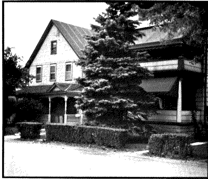
Photo No. 15. Homes on School Street near mile 2.25 which are affected by sewer backup when sanitary sewer manholes are covered.
