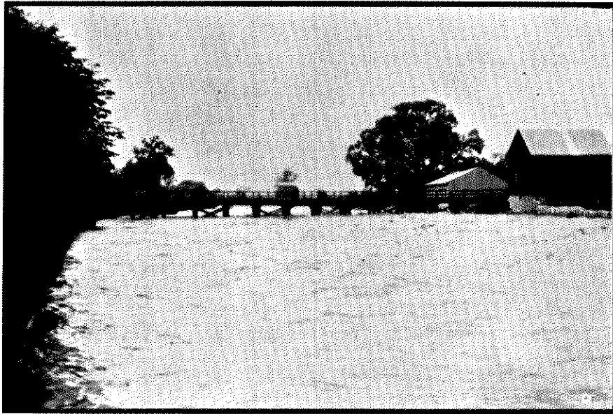
Photo No. 1. Looking downstream at temporary bridge used during construction of Union Road bridge during the flood of the summer of 1928.
