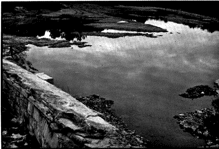
Photo No. 22. Looking upstream from Blossom Dam. Photo shows removal of gravel bar at upper left and shows riprap on bank at upper right which was placed by the Soil Conservation Service.
