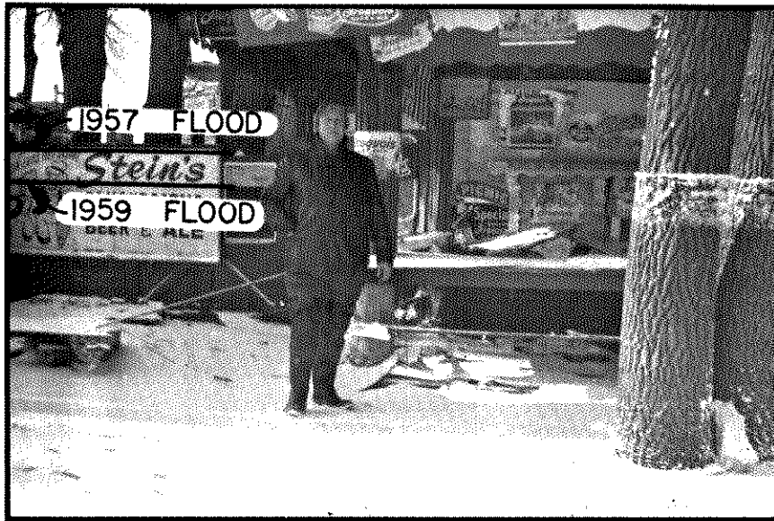
Photo No. 9. Ice lines indicate January 1959 flood elevation at Huppertz Grove, Collins Avenue. Near mile 0.15.
