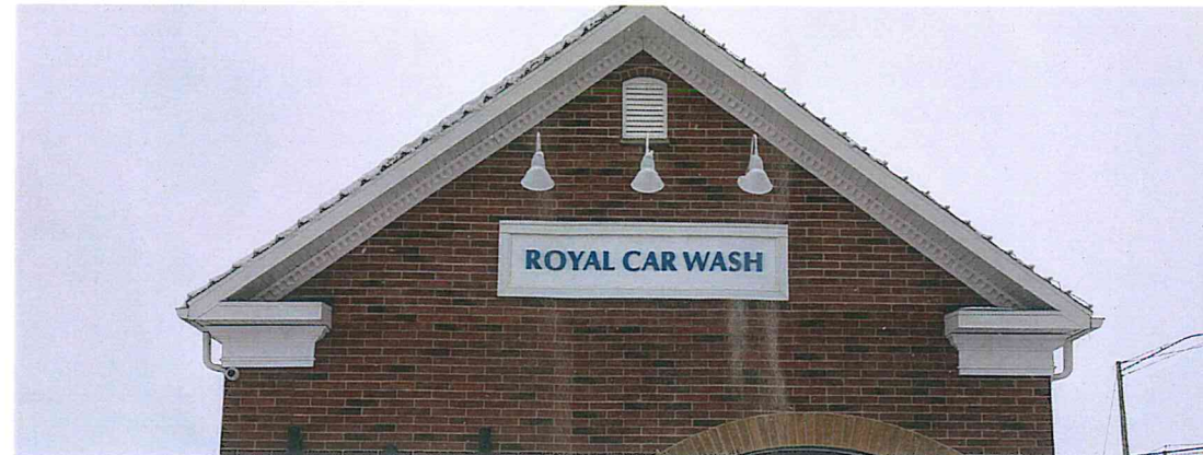
BUILDING MOUNTED SIGNAGE (x2) ABOVE TUNNEL ENTRANCE/EXIT
