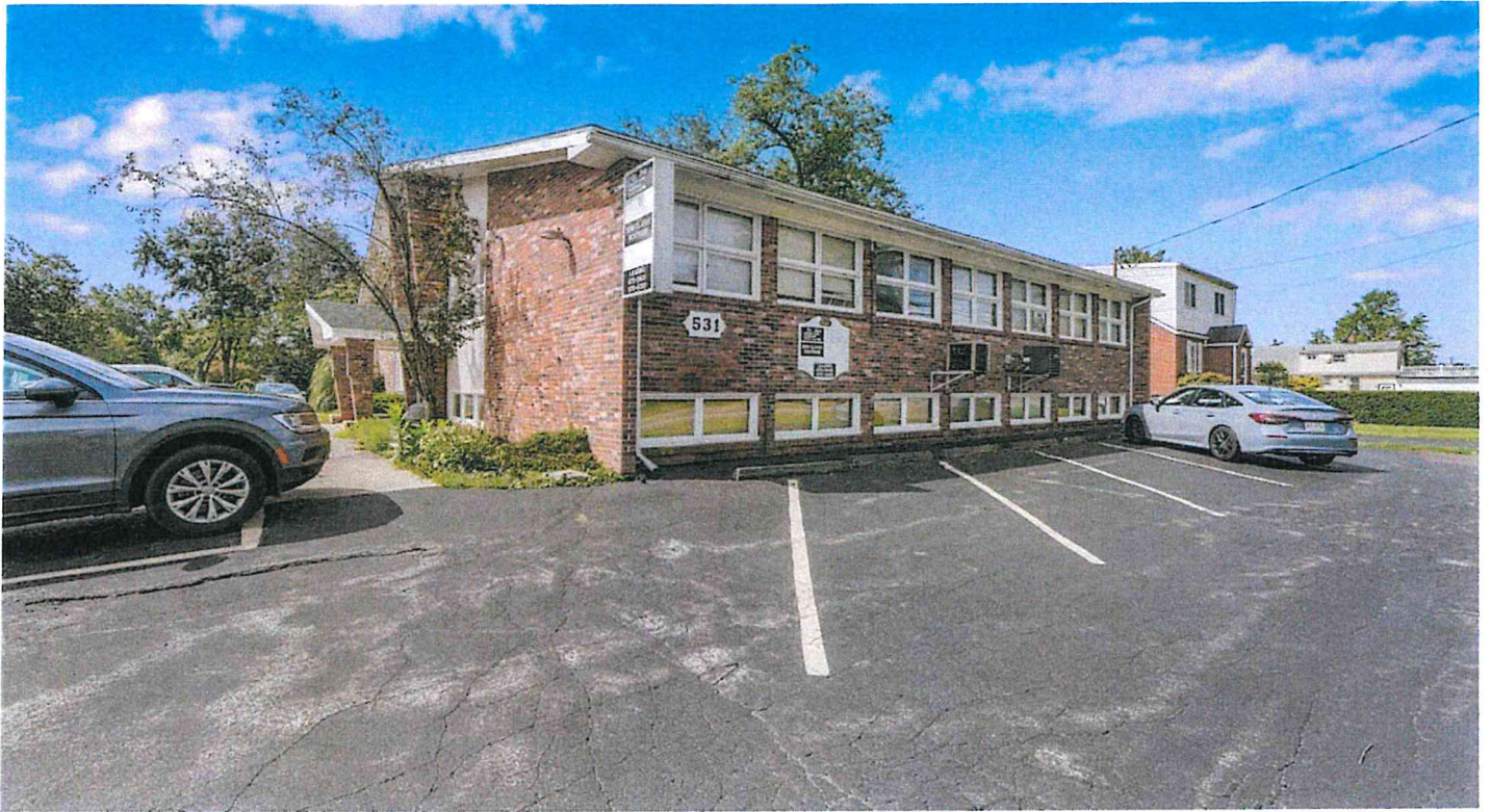
Photo of Existing Building From intersection of Center Road and Florence Avenue
