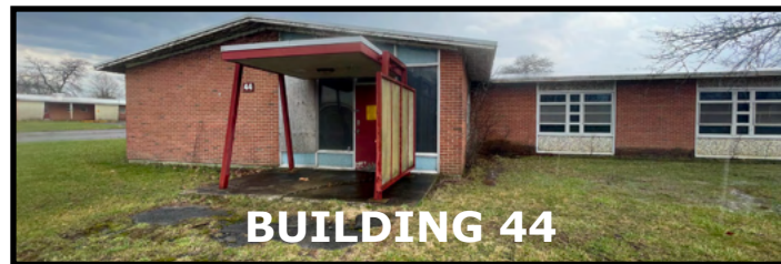
Figure 2.4: Former Dorm Building
