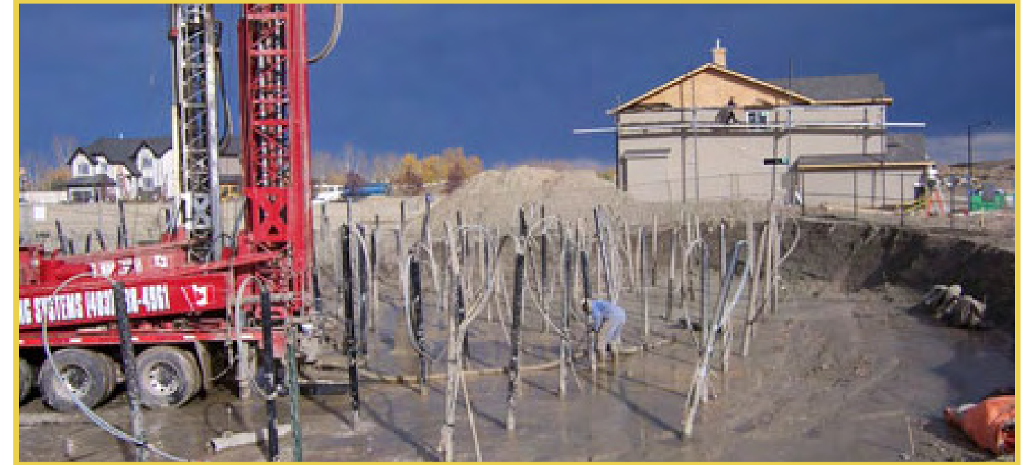
Figure 3.1: BTES System Installation
