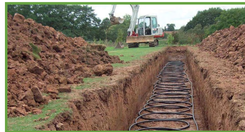
Figure 4.4: Horizontal Geothermal Installation
