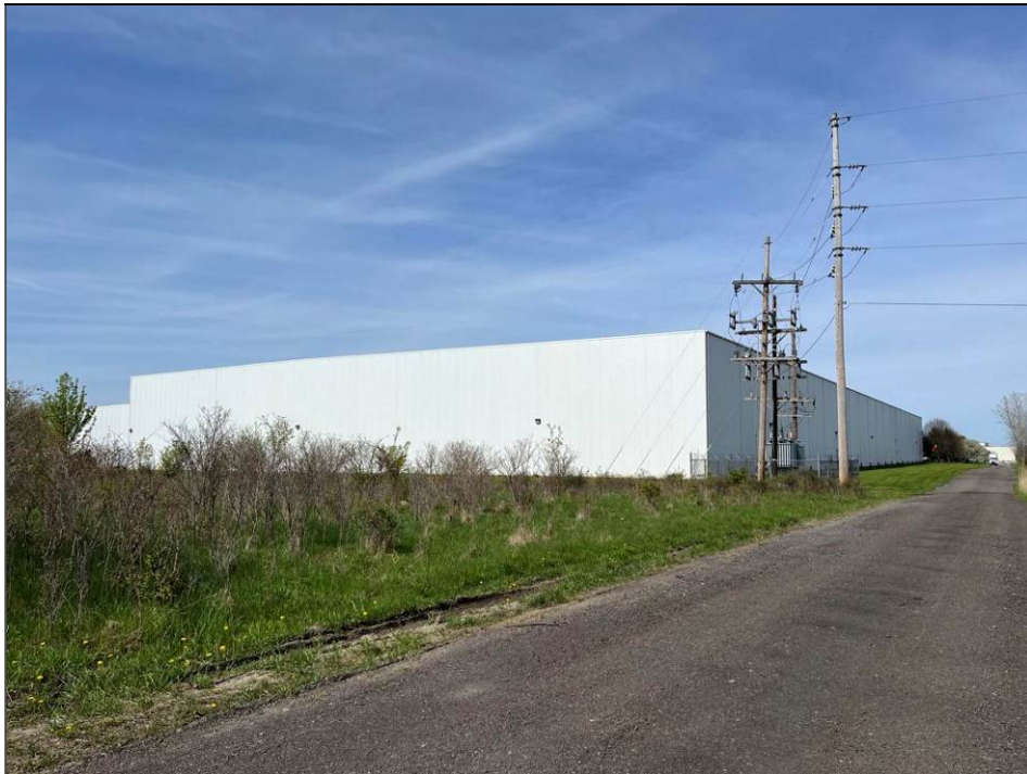
Photograph 32. Access road and general vicinity south of the APE, looking west / southwest.
